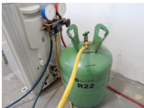
When charging R22 gas, bottle to be upright
