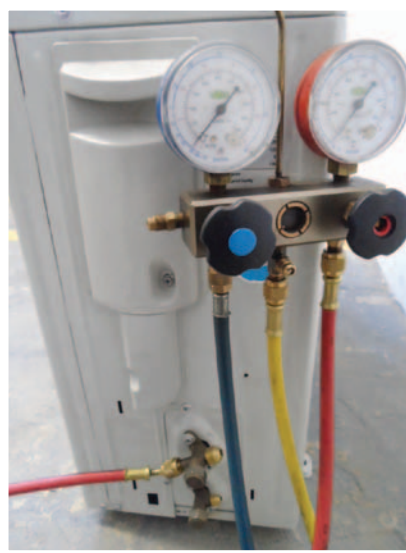
Heating pressure check: fit red hose while unit running on cooling, then switch unit to heating
