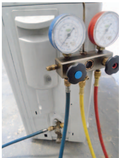
Cooling pressure check: blue hose fitted to suction port
