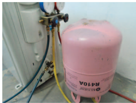
When charging R410A gas, bottle to be upside down
